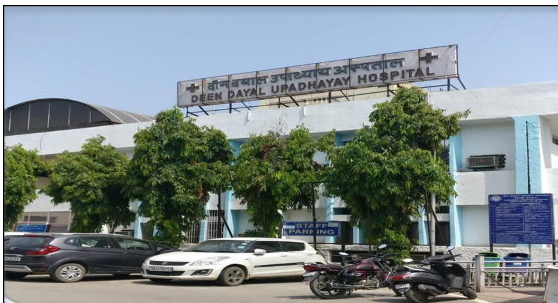
DDU Hospital Main Entrance
