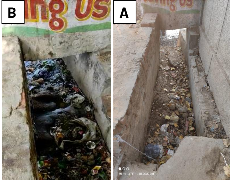
Mongolpuri X- block Drain
