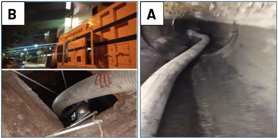
Keshopur STP Bhera enclave near VR hotel
