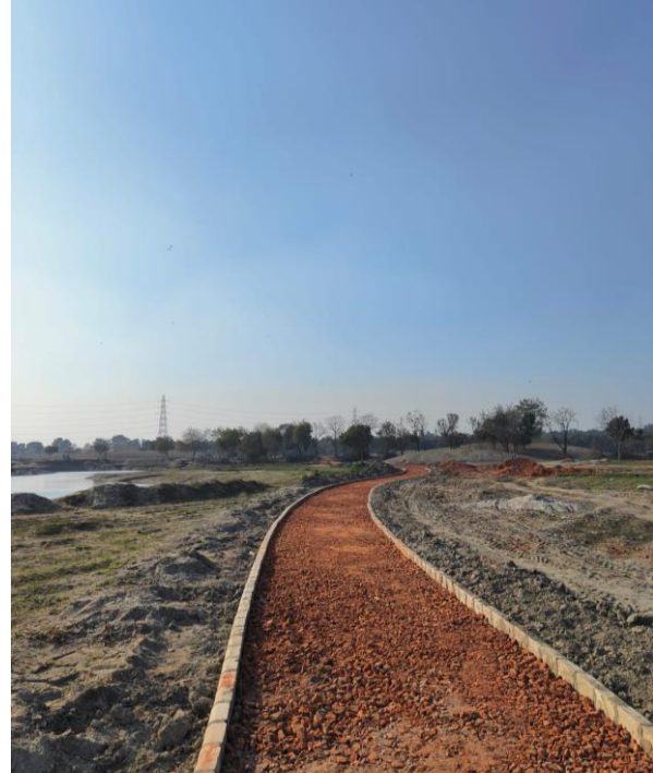
Pathways and parking being developed
