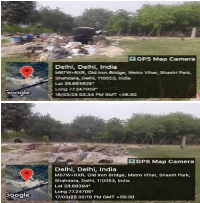
07 - Illegal Bhattis Dismantled
