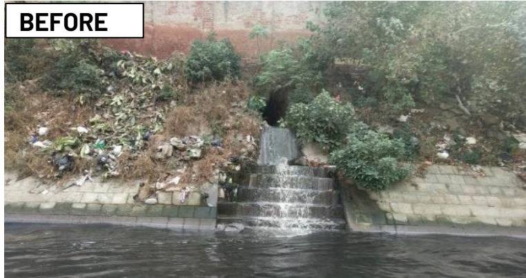
Shakti Nagar Nagar Drain-3 Right Bank 51975m
