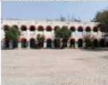
Educational Facility at Ghoga Village
