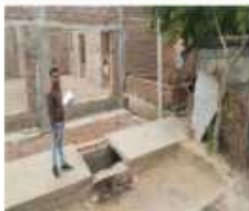
Drainage Facility in the Study Area, JJ Colony
