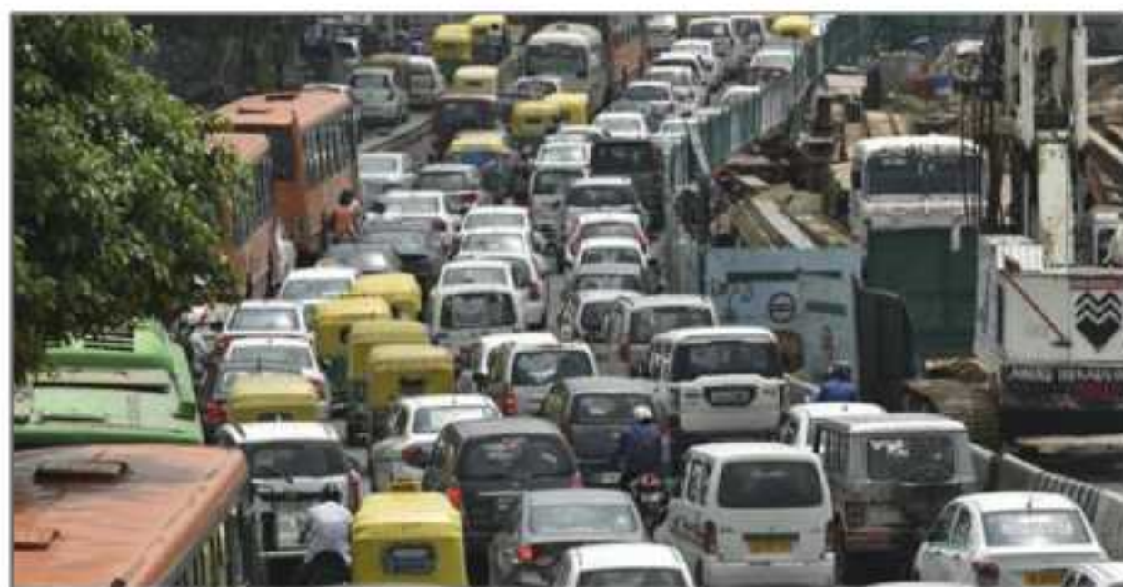
Another view of the inner Ring road in South Extension where restricted space for vehicular traffic movement has been further narrowed by ongoing metro construction works.
