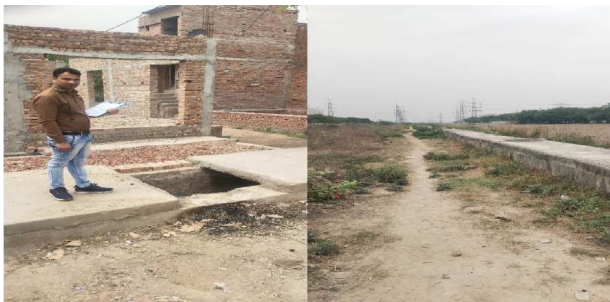
Closed Drainage facility in the study area
