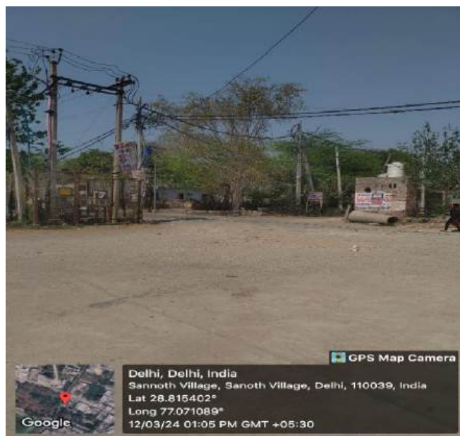
Figure 3.44: Power Supply Facilities
