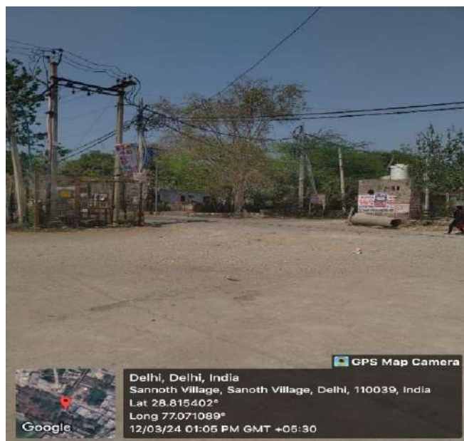
Figure 3.44: Power Supply Facilities
