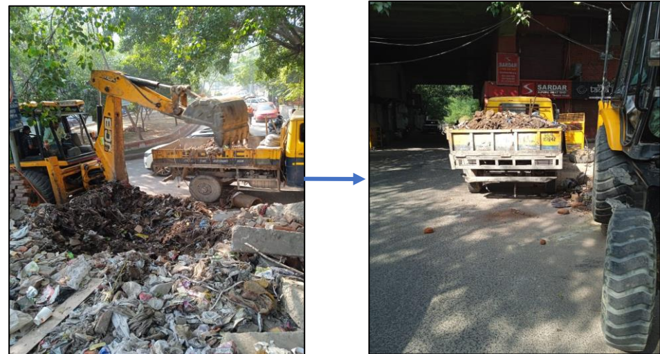
MSW lifted along the tracks in Central zone
