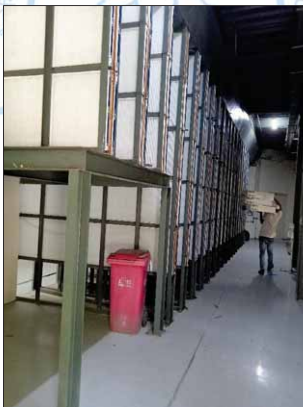
Figure 151. Fine filter installation in the filter bank.
