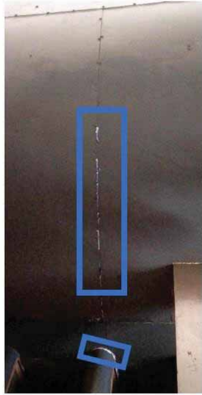
Figure 16. Structural joint sealing using silicon for arresting the system leaks.
