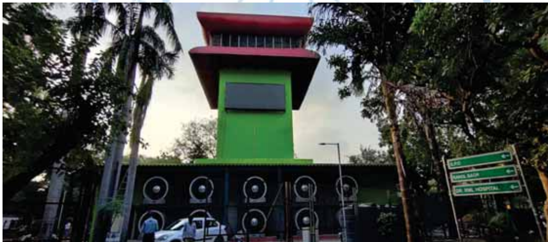
Figure 6. MSACS site view after completion of the construction.
