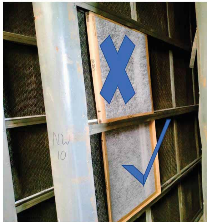
Figure 8. Pre-filter installation.
