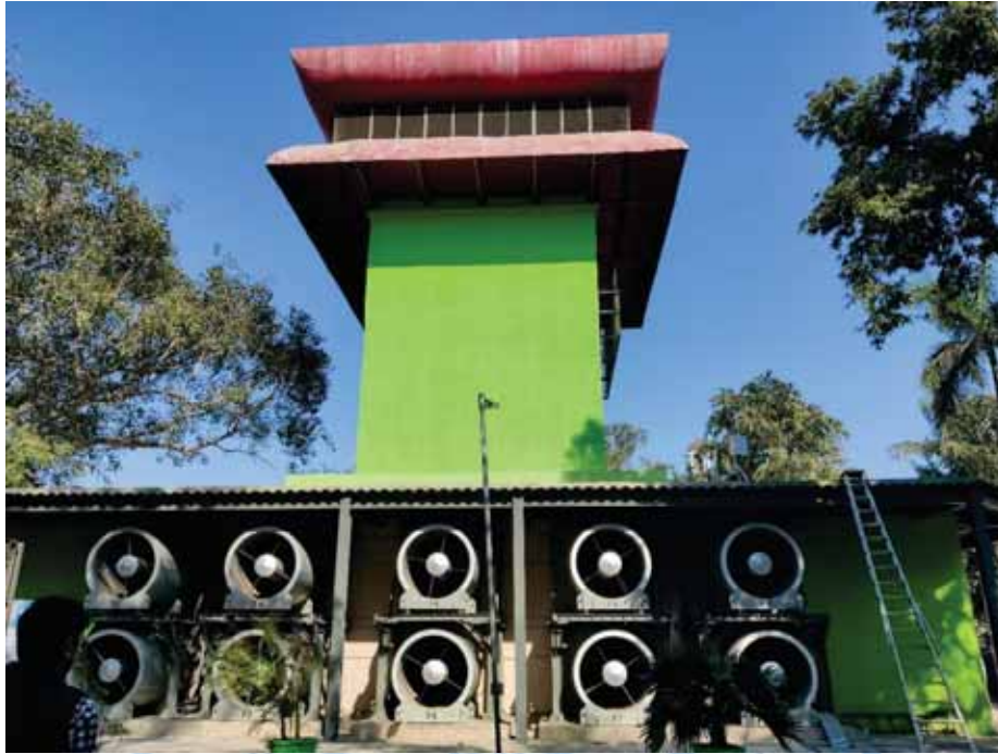
Figure 5. MSACS constructed at Connaught Place, Delhi.
