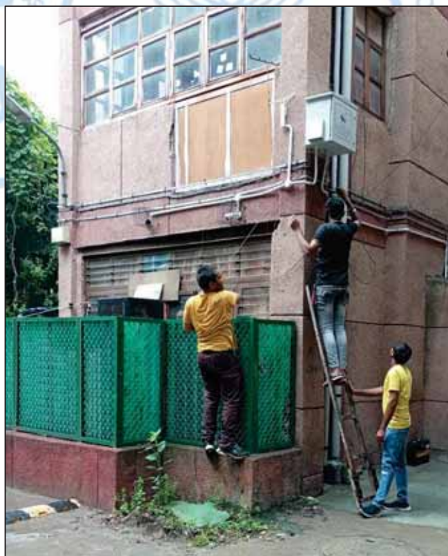
Figure 166. Fixed LCS Maintenance.
