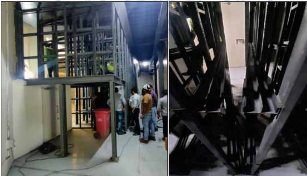
Figure 149. Filter frame assembly cleaning prior to fresh filters placement.
