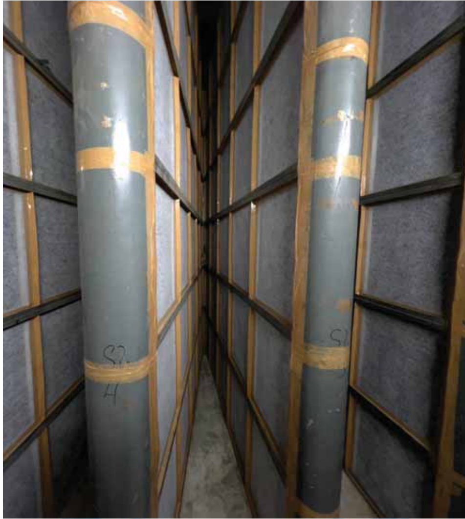
Figure 15. Pre-filters are joined side by side using good-quality adhesive tapes to arrest the leaks/gaps between the filters.
