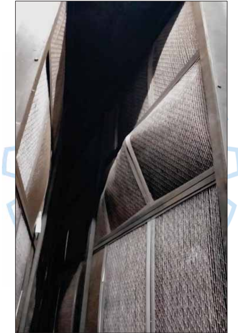
Figure 116. Bending of the fine filter inside the MSACS.
