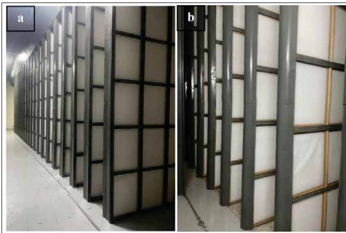
Figure 152. (a) Fine and (b) Pre-filter installation work completed.
